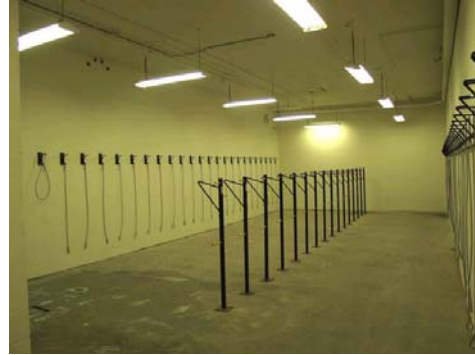
Bicycle Storage Room at VITP
