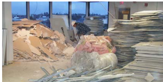
Construction waste was separated and recycled during the VITP construction.
