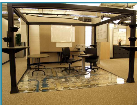
Raised floor with underfloor cabling
